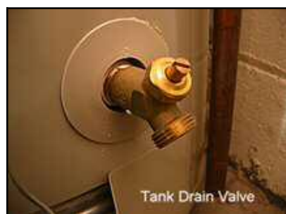
Figure 7.19: Drain Faucet – The drain faucet on a hot water heater. Note that it threaded to couple a garden hose to it for draining purposes. Source: internet – [file:\DrainFaucet[40].jpg].
