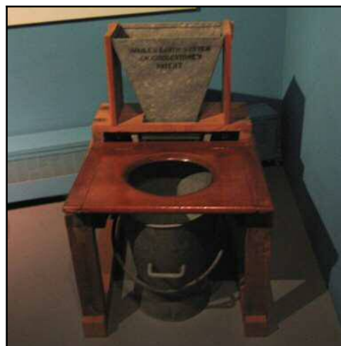
Figure 8.5: Dry Earth Toilet – Patented in 1860 by Henry Moule, the dry earth toilet was the forerunner of WAG bag and composting toilet. Source: internet – [file:\DryEarthToilet[53].jpg].
