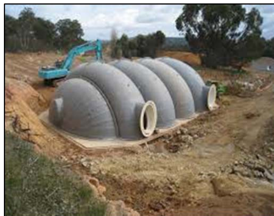
Figure 11.22: Fiberglass Bunker – Providing scale, note the large shovel in the background. When complete, the entire unit will be buried. Source: Internet – [file:\ModularFiberglassBunker01[70].jpg].
