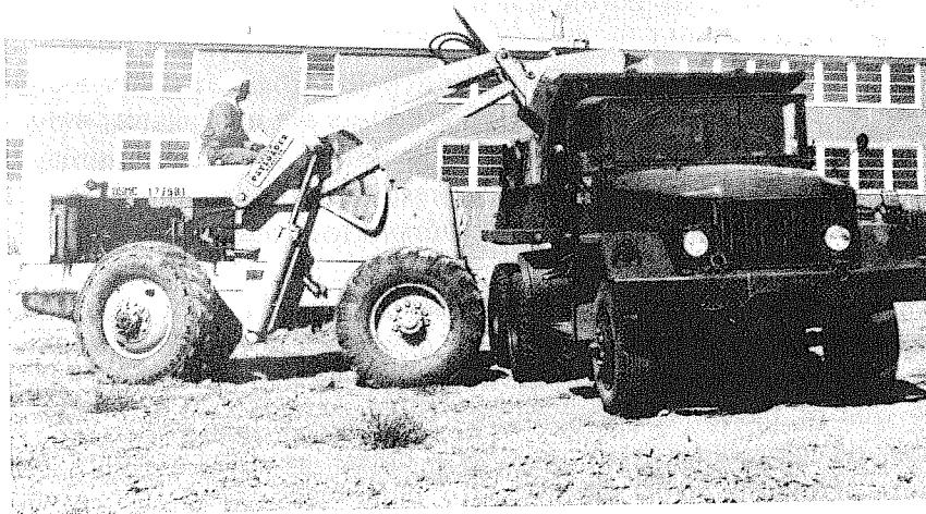
Removing fallout from an unpaved area.
