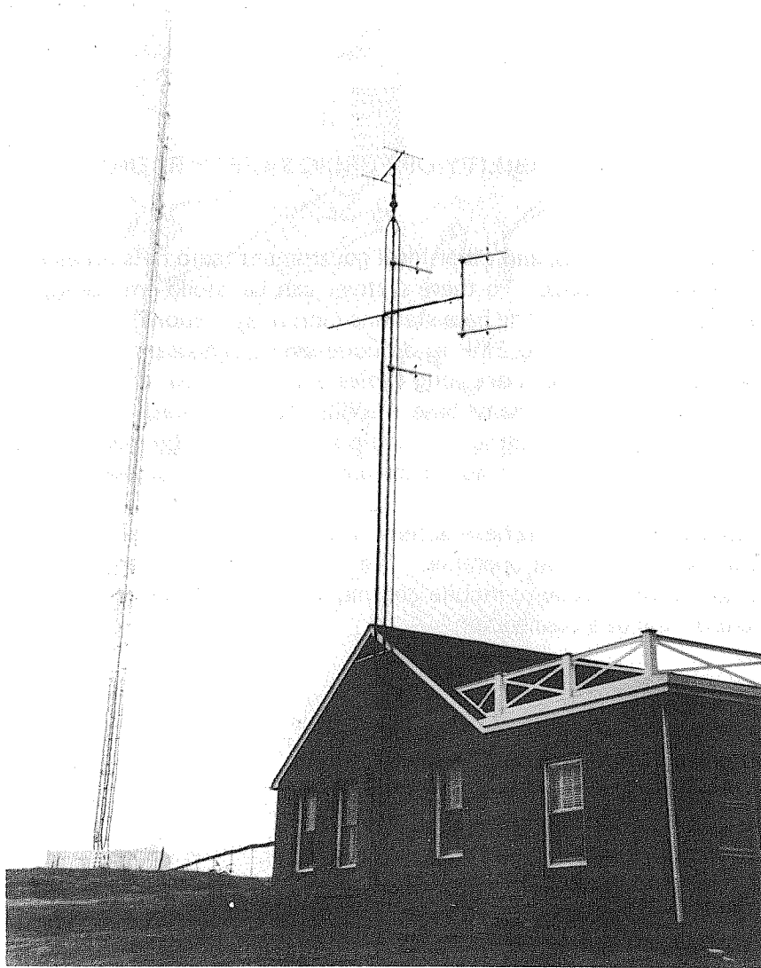
AM BROADCAST STATION ANTENNA AND TRANSMITTER BUILDING
