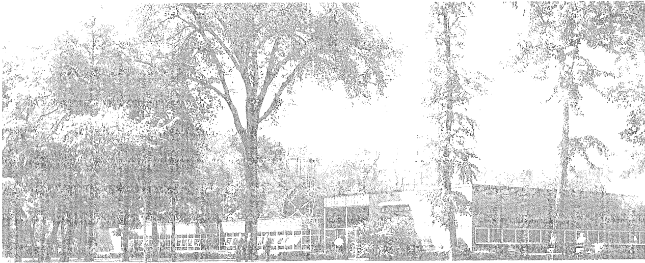
The Detroit civil defense building, built in 1954, is used for administrative purposes. The EOC is directly below. Note radio communications tower.
