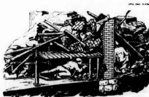
Fig. 131. Providing access into the rubble.
