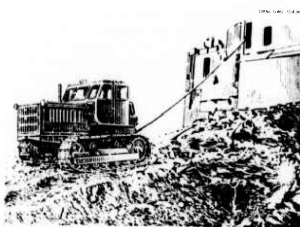
Fig. 134. Demolishing an unstable structure with a tractor.
