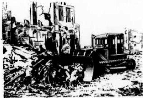
Fig. 122. Clearing a passage with a bulldozer.
