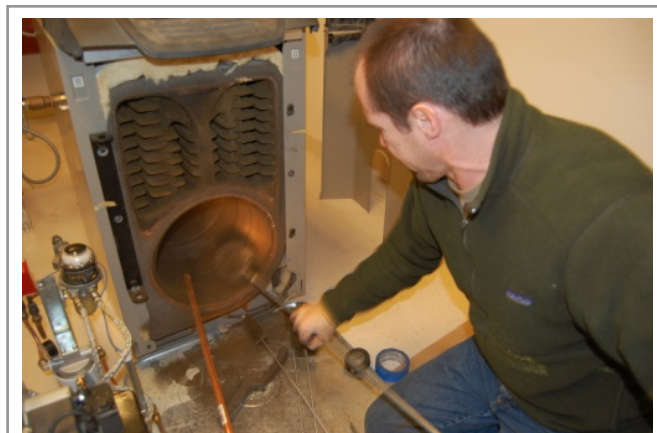
A contractor cleans and inspects a boiler
