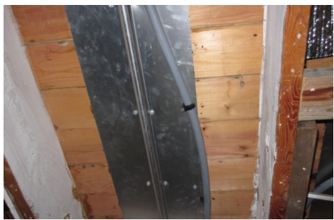
This "staple up" radiant floor system uses metal connectors to help distribute heat to the floor. View from basement.
