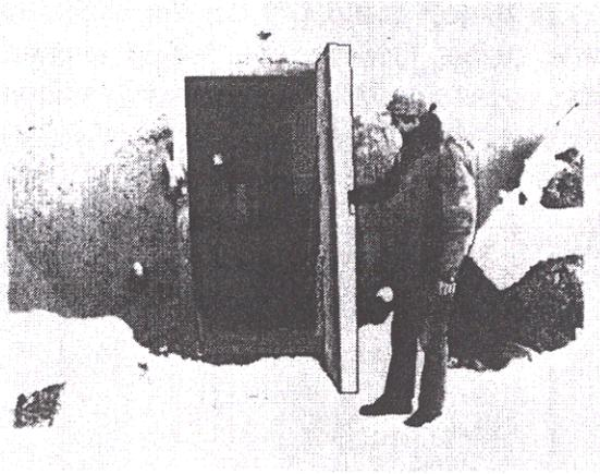
Doors opening to the inside allow occupants to open them even when blocked by accumulated rubble. These style doors are more difficult to construct because the overpressure is carried by dogs or pins which extend from the door into the door frame. These dogs transfer the overpressure to the door frame. Therefore, inwardly opening doors need to be small.
