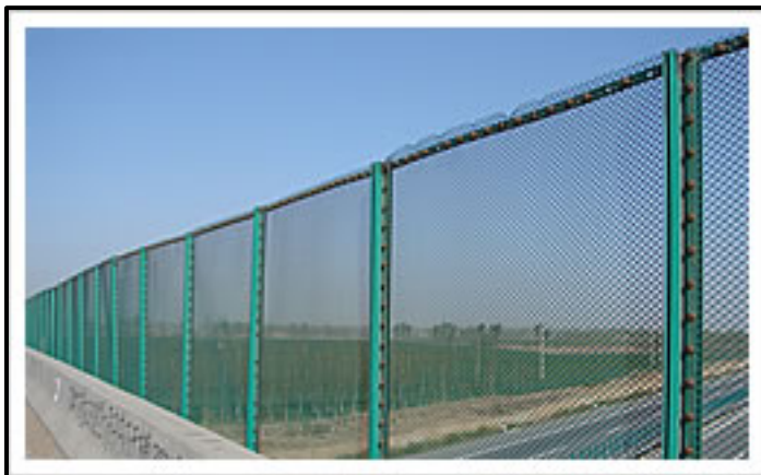
Figure 2-4: Expanded Metal Fence
