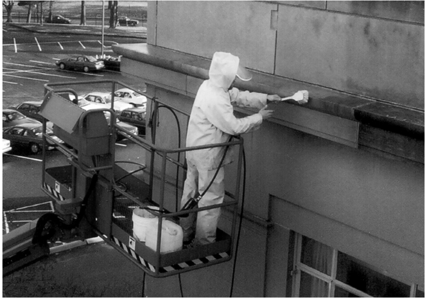
A worker scrubs and removes softened soil from the water-soaked limestone façade.
