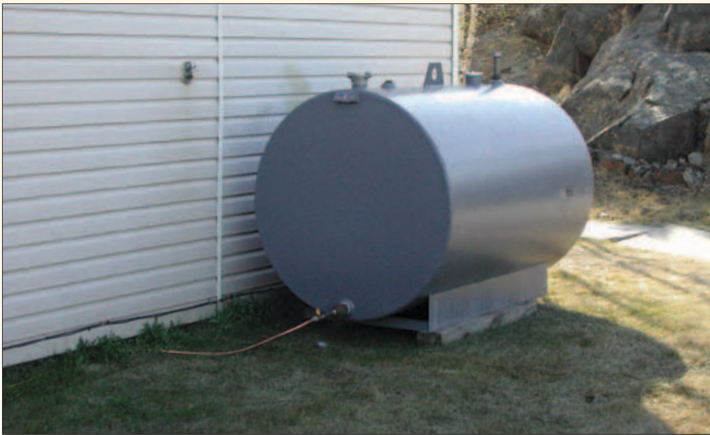
Double-wall steel heating oil tank.
