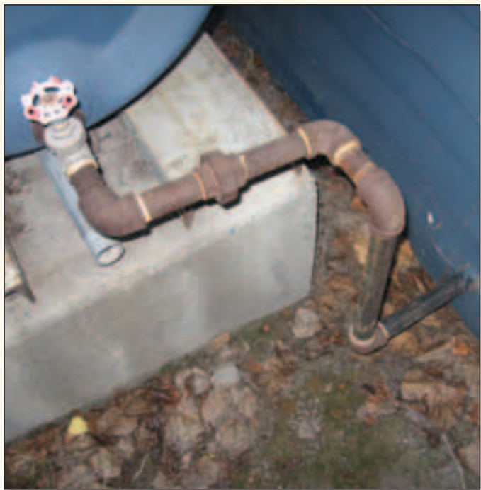
This type of fuel line is called a swing joint, which accounts for tank movement.
