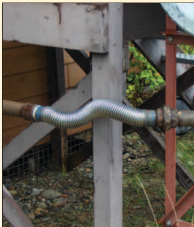
This flex connector is out of alignment.
