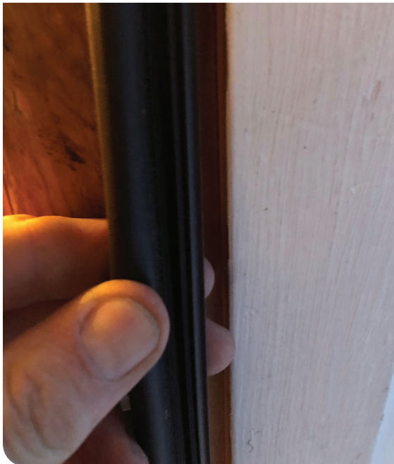
Press the new weather-stripping into the groove in the door frame
