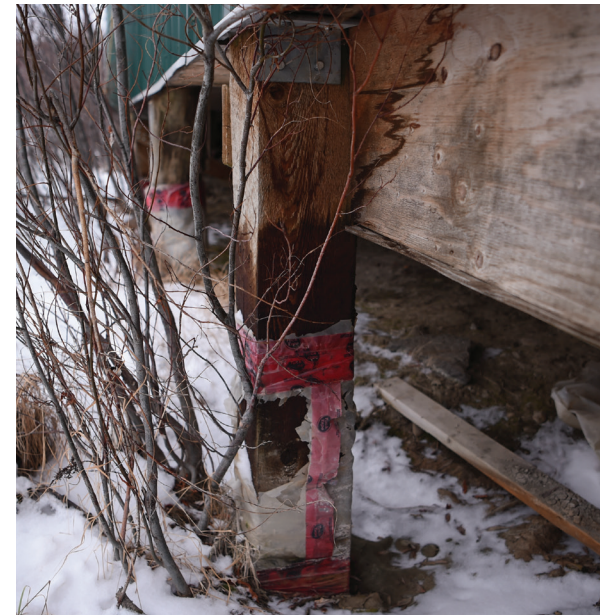
Mould and rust can cause damage to foundation footings
