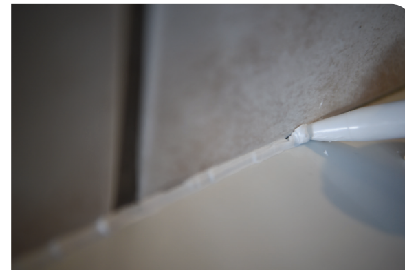
Caulk floor at base of tub
