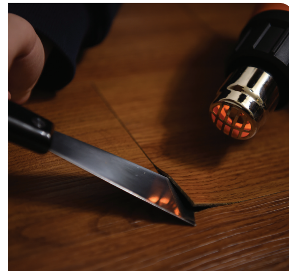
Lift floor tile with heat & putty knife
