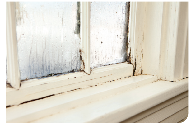
Damage caused by condensation on windows.
