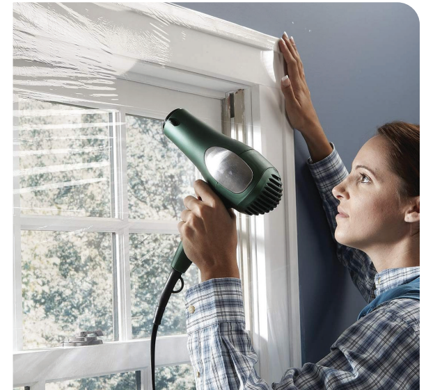
Installing plastic window film
