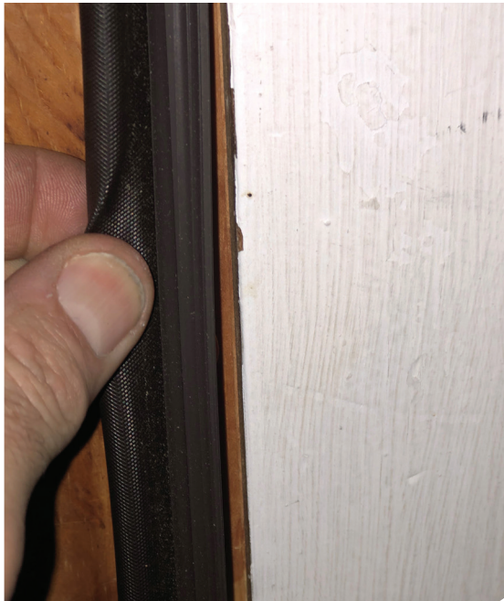
New weather-stripping installed in doorjamb
