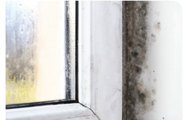
Mould buildup on inside of window frame.
