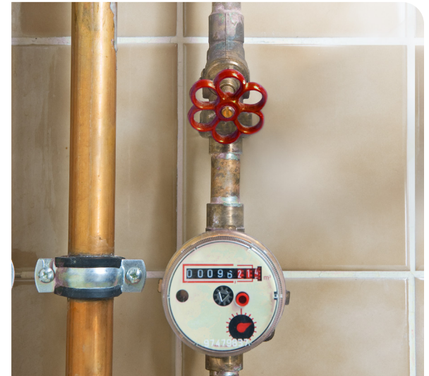
Main water turn off valve. Also note the water meter on the main line.
