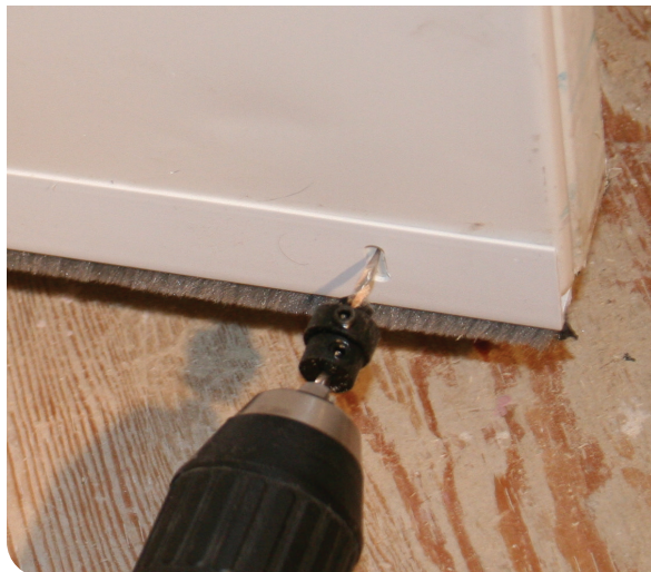
Drill holes for screws in door
