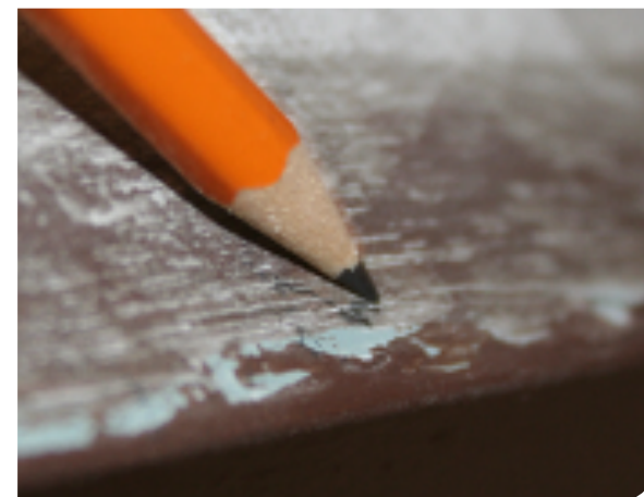
Remove built up paint from door
