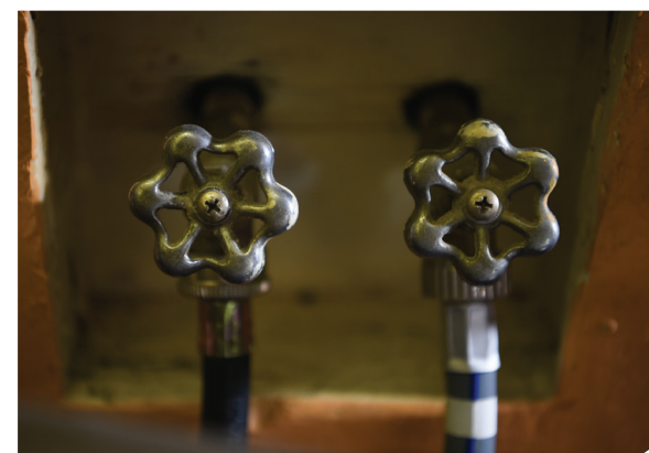
Hot and cold water shut off valves
