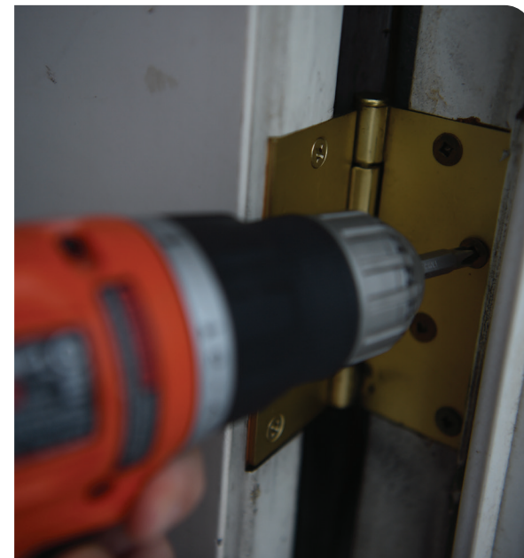
Install a 2 ½" screw in hinge
