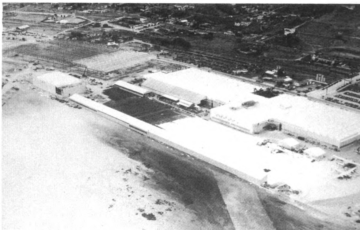
Figure 24—A type of factory construction most difficult to black-out. {Note glare from sawtooth glass roofs.}
