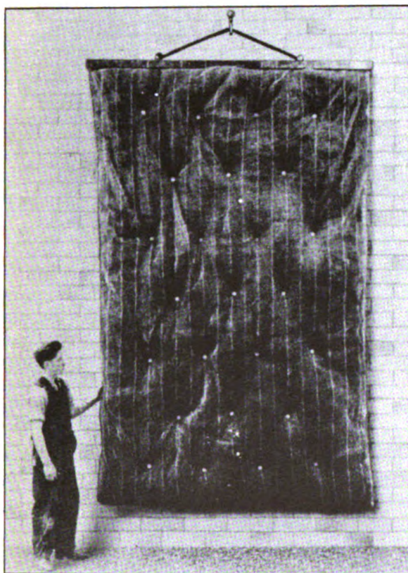
Figure 25—Typical metal wool mattress for covering window.
