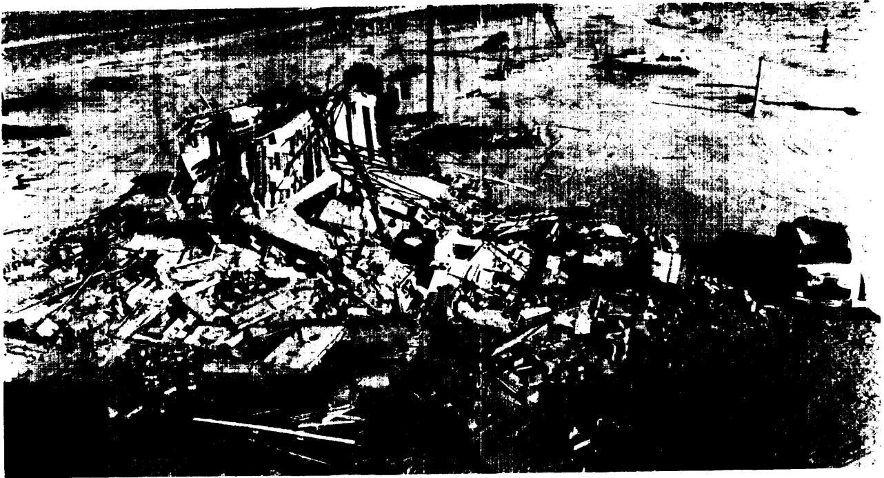
Damage to unreinforced brick house (5-psi overpressure)
