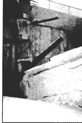
Above and left, the Queens parking garage collapse. In photo at left, note where corbel used to sit. It was not reinforced. Remaining corbels are holding garage floor in photo above.
