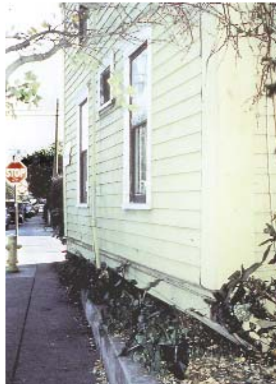
Cripple wall foundation failure, Northridge, Calif.
