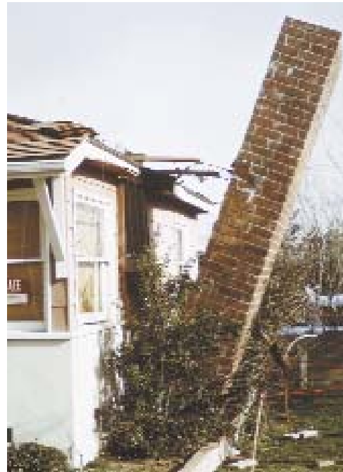
Chimney damage, San Fernando, Calif.
