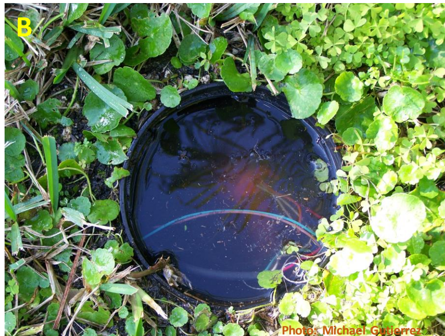
Figure 23. Picture A shows a wire connection, capped with a common electric connector, before inserting it into the waterproof grease cap connector. The waterproof grease caps are used to protect the connection between the probe wires and the extension wires coming from the controller or valve, encased in a valve-box. Picture B shows waterproof grease cap connectors completely submerged in water.
