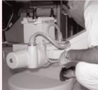
Clean and decontaminate the worksite.
