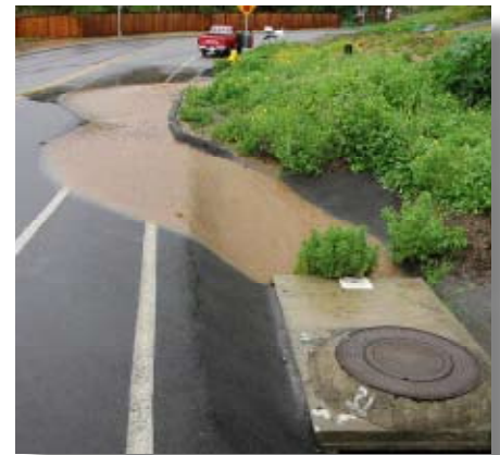
Polluted stormwater runoff flowing into a storm drain.
