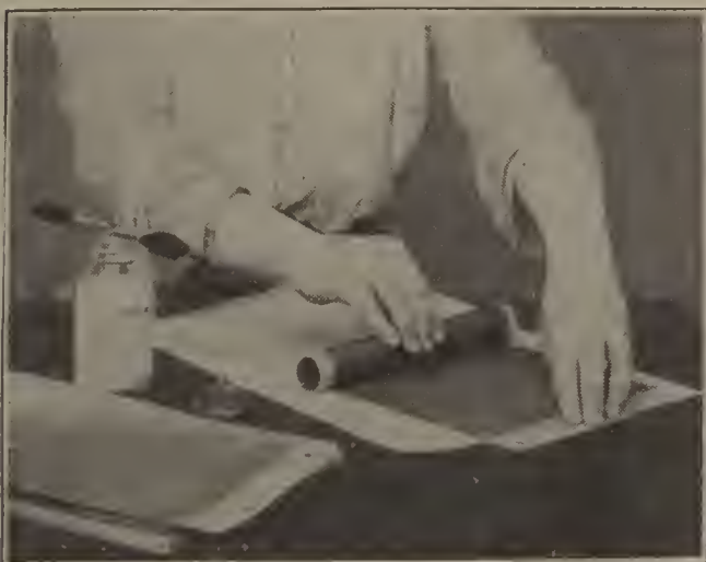
Method of smoothly relaying the Stencil Sheet
