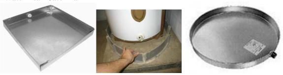
A water heater tank should be installed inside a pan in locations in a dwelling where a leak from the tank could cause damage to the structure or property. The pan is intended to catch water leaks from the tank or associated connections, or condensate from the tank.
